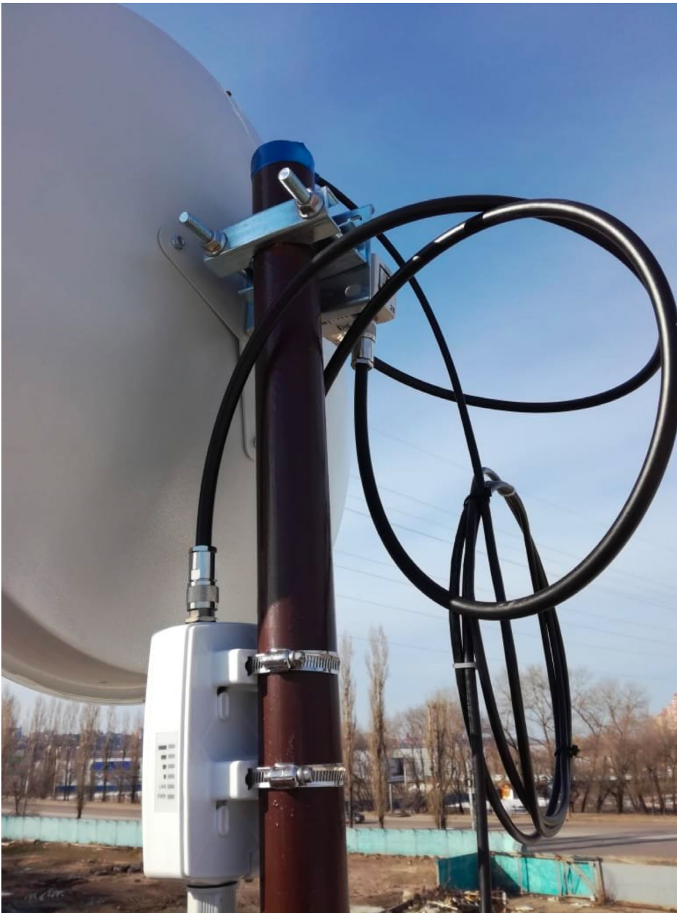
Image | LigoDLB 6ac with External Dish Antenna
